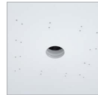
Line up remaining drywall
