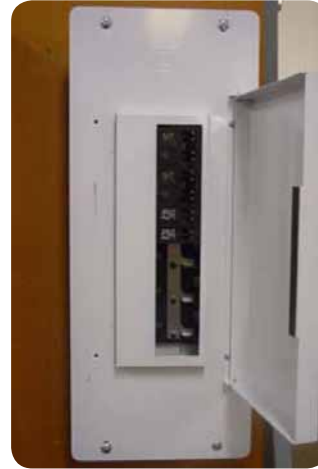
Step #3 Install New HFLCI
