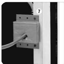
The bracket mounts directly onto the stud.
