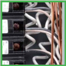
Pigtail Neutral Connections
